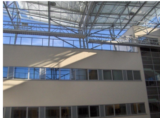
Fig. 3. Atrium-type building (B) with opened to the outdoor air cap between the floor and the walls
