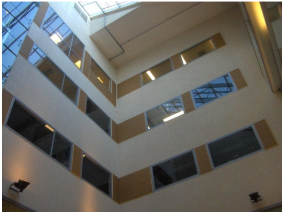
Fig. 2. Atrium-type building (A) that is tightly covered with glass roof. Only the workrooms beginning the 4th floor are sun lighted
