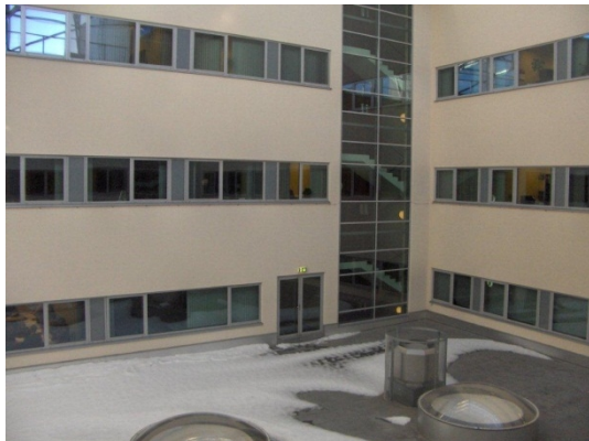
Fig. 4. As there is a slot between the roof and walls in the building (B), the snow is falling on the atrium floor in winter
